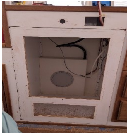
The Old refrigerator fit into the upper opening. Note the Cutout for the New refrigerator.
